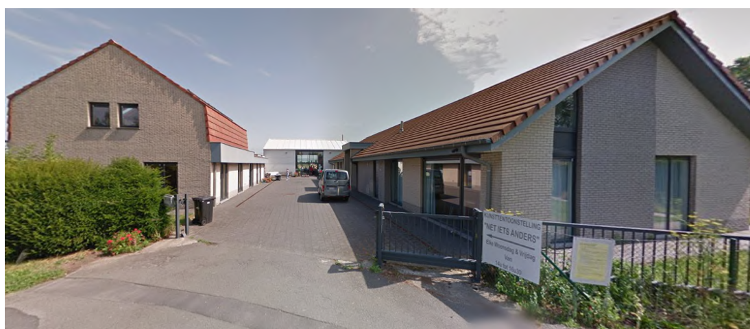
Figuur 5 – Site De Bollaard (bron: Google Streetview)
